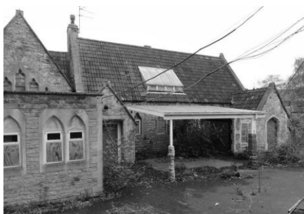
Derelict Bath Hill School (Photo- Don Ogg)
